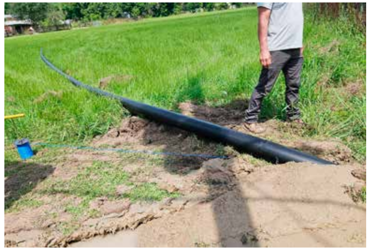
Crews begin the installation of a new 6-inch water line along La. Hwy. 77.
