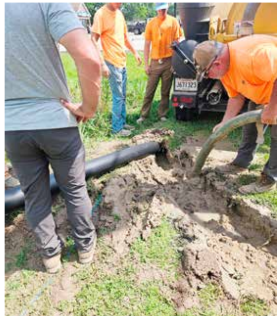
Crews begin the installation of a new 6-inch water line along La. Hwy. 77.
