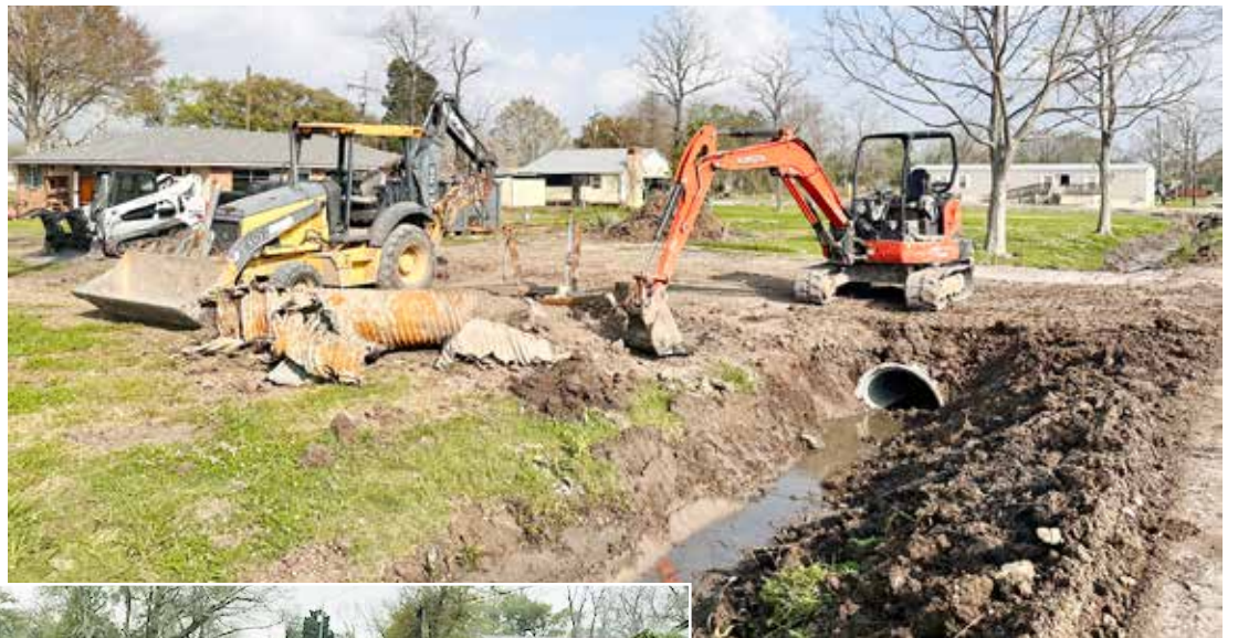
The photo above shows one of the old culverts and the new drainage culvert. The photo at right shows regraded ditches to improve drainage.
