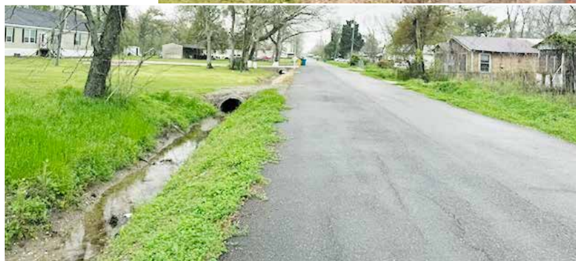
The photo above shows one of the old culverts and the new drainage culvert. The photo at right shows regraded ditches to improve drainage.
