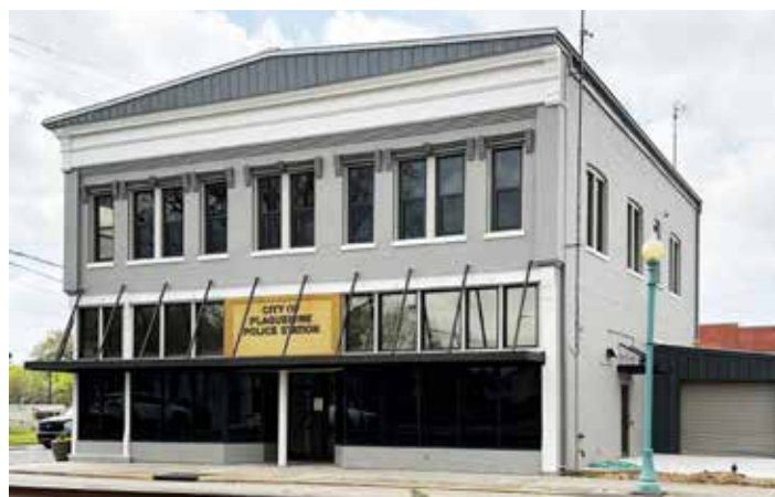
Police Station repainting underway.
