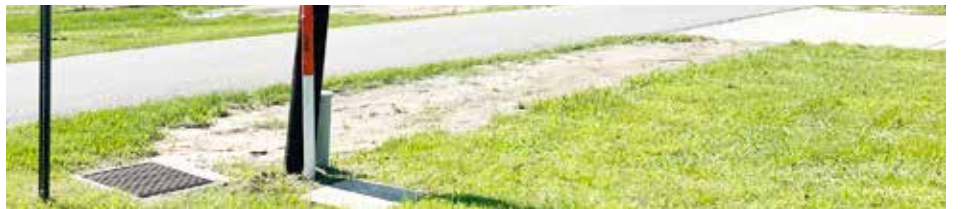
Completed larger drainage culverts on Lions Street.
